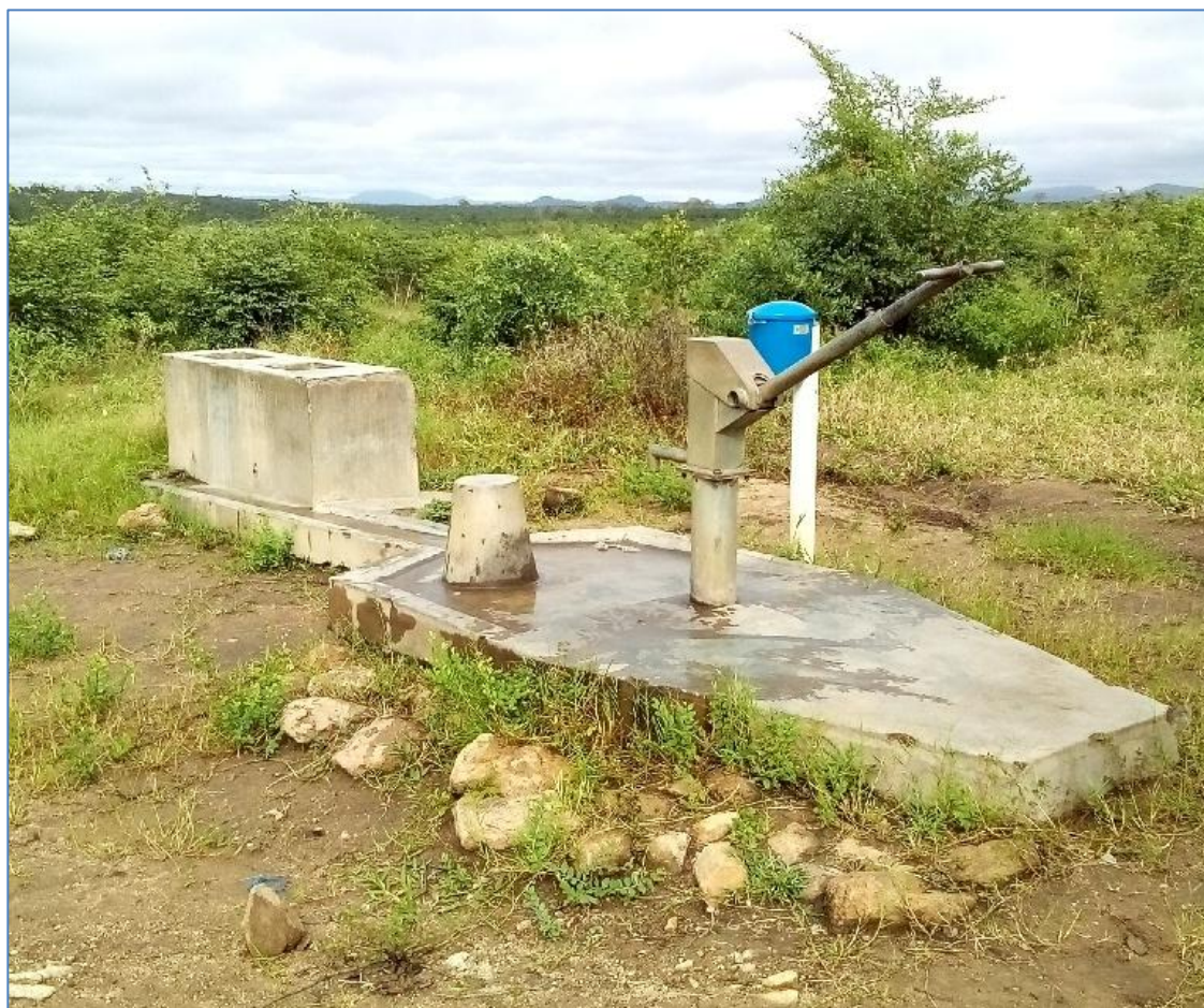
Figure 33: Community Borehole affected in Nkhwali Village
